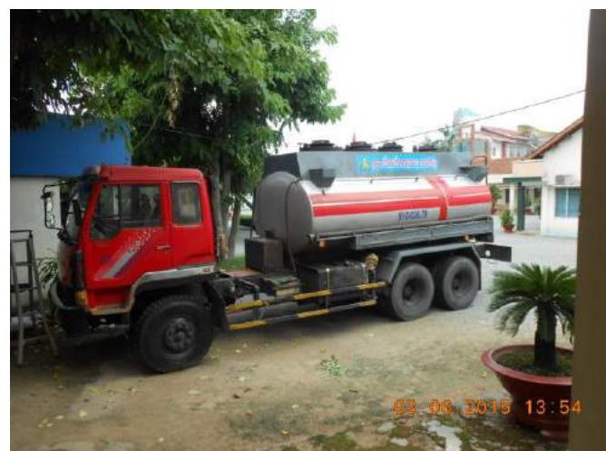
Dustproof water tank is used to water the construction area.
