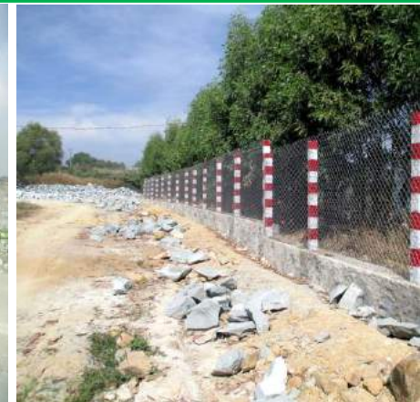
Building the safety fence around the pit banks - planting trees to prevent dust emissions
